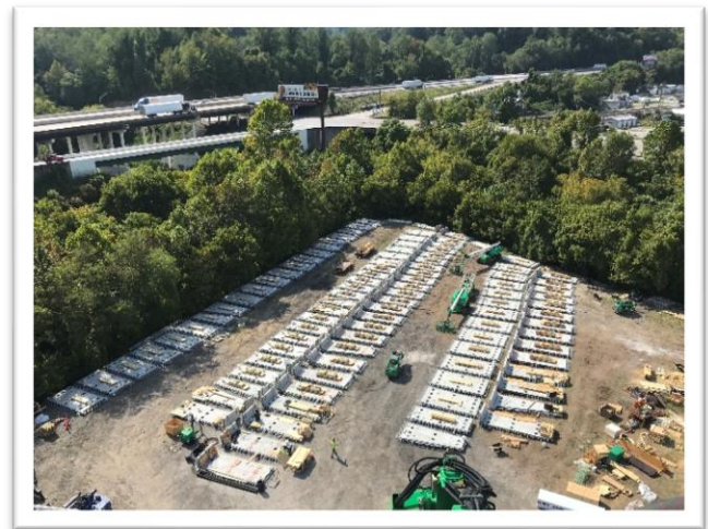
Off-Site Staging of the Pre-Cast Deck Panels
