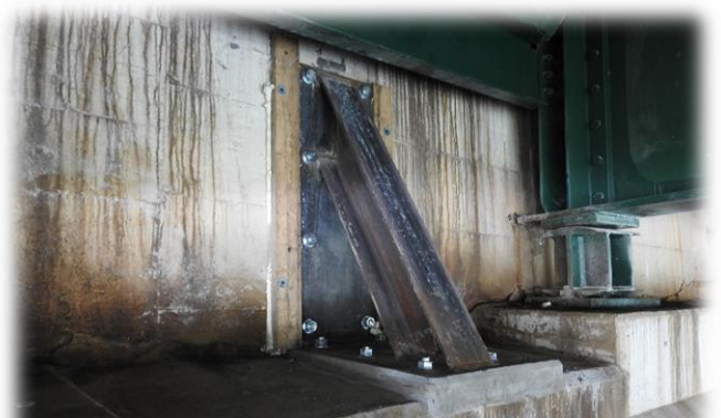
3076N S, Abutment Counterfort Retrofit
