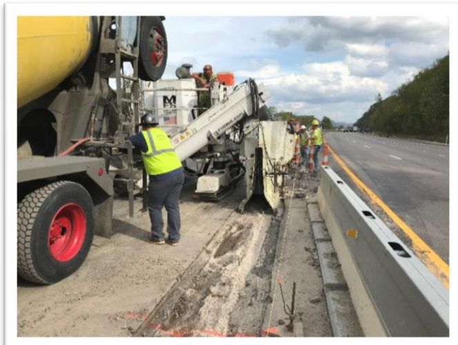
Slip Forming Median Wall
