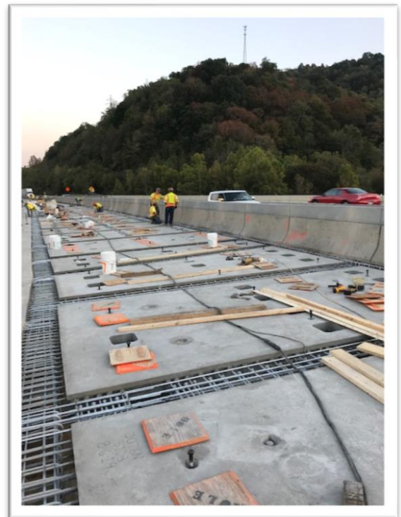
Pre-Cast Deck Panels in Place
