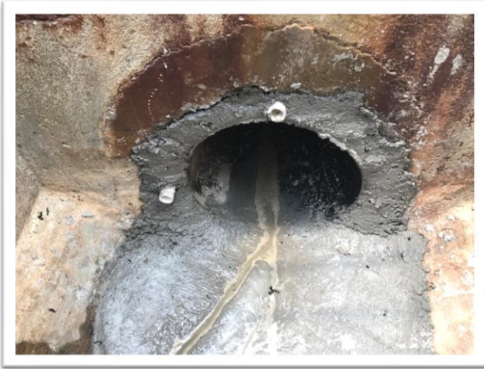
Grouted Dump Rock Gutter
