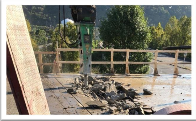
Demolition of the Existing Bridge
