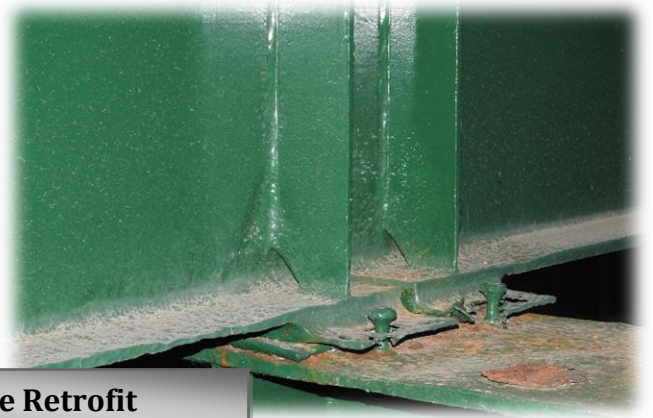
Bridge 3038N Bearing Retrofit
