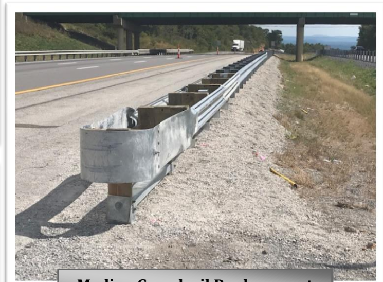
Median Guardrail Replacement
