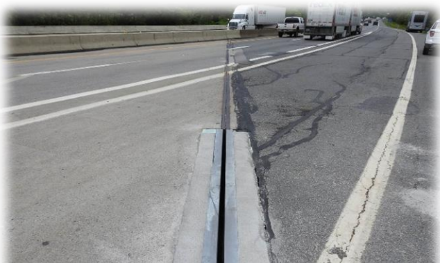
Bridge 3065S Deck Joint Replacement
