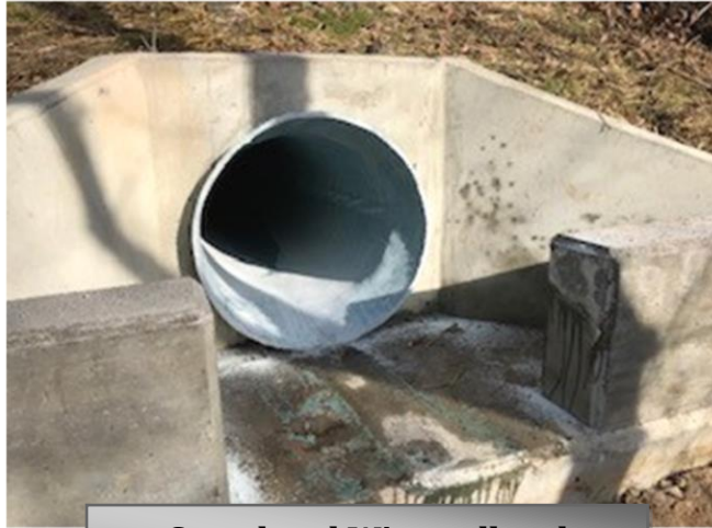
Completed Wingwall and Culvert Liner
