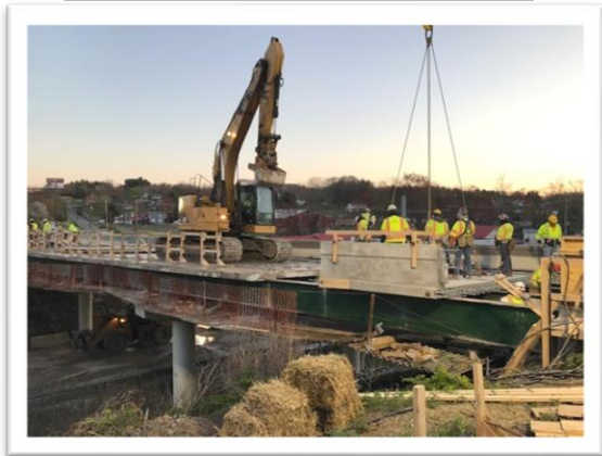
Deck Removal and Placement of Pre-Cast
