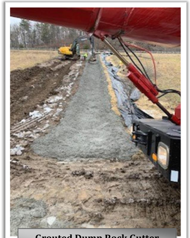
Grouted Dump Rock Gutter Installation
