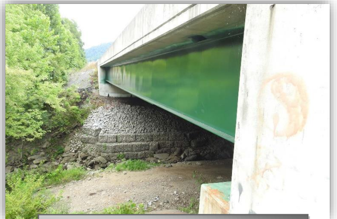
Bridge 3083 Fascia Steelwork
