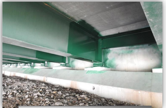
Bridge 3070 Abutment Steelwork
