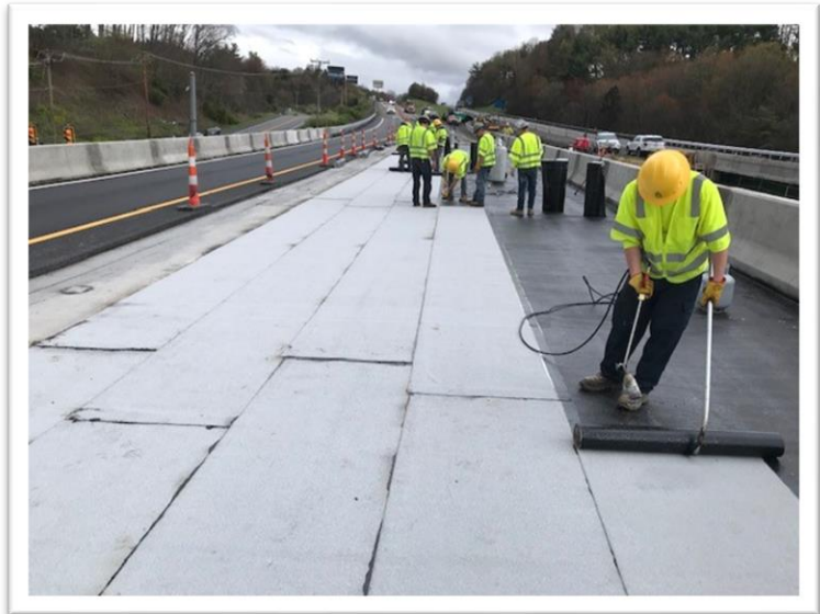
Waterproof Membrane Installation
