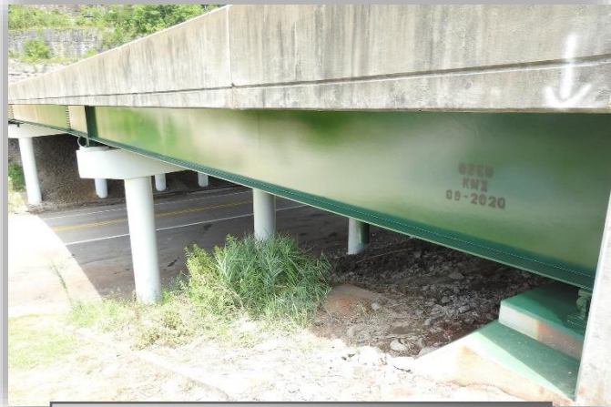
Bridge 3070 Fascia Steelwork
