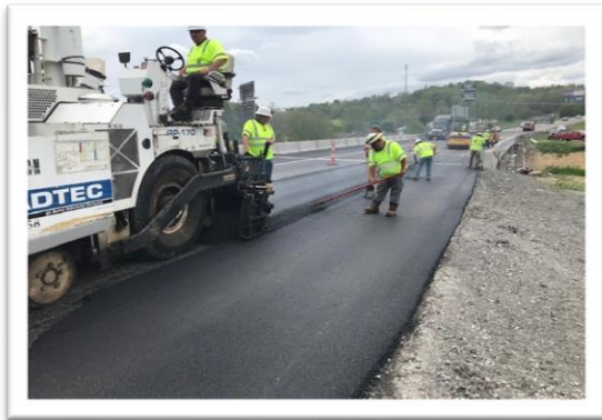
Bridge Departure Paving
