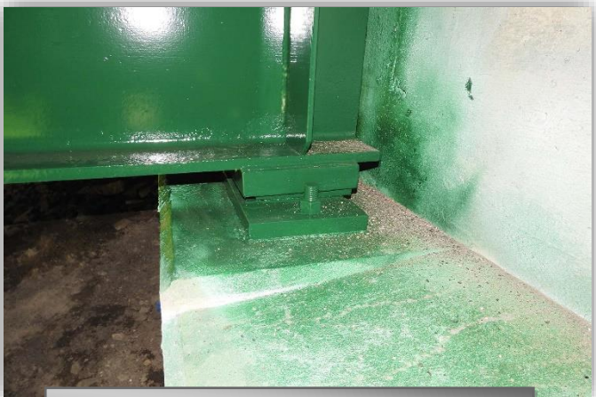
Bridge 3080 Fascia Steelwork
