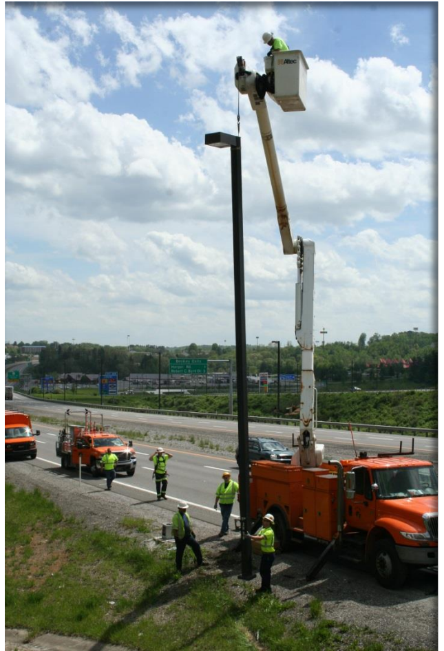
Roadway Light Pole Repair
