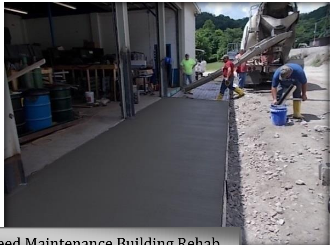
Reed Maintenance Building Rehab
