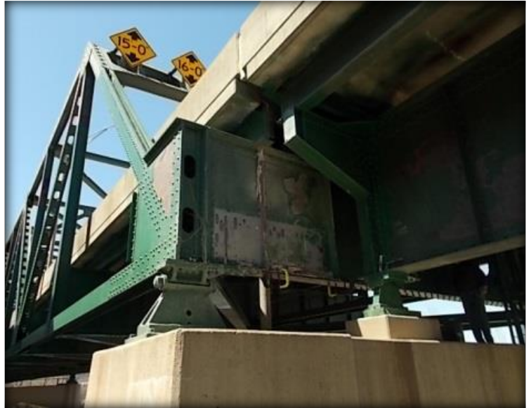
Yeager SB Section Loss Retrofit at Pier 6
