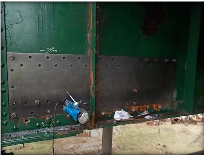
Yeager SB Section Loss Retrofit at Pier 6
