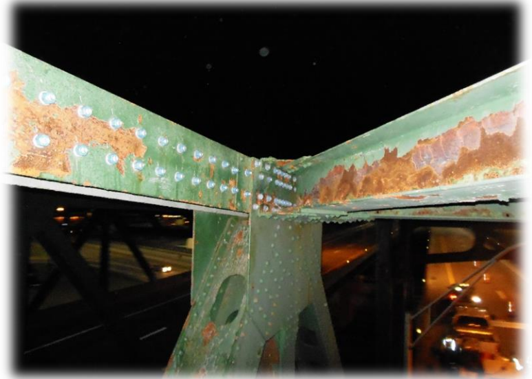
Longitudinal Angles Installed on the Top Chord of South Yeager Bridge
