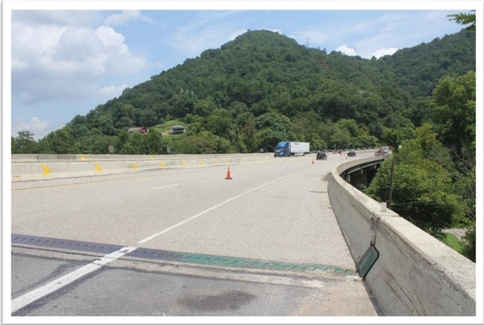
Bridge Deck Overlay with Non-Skid Surface
