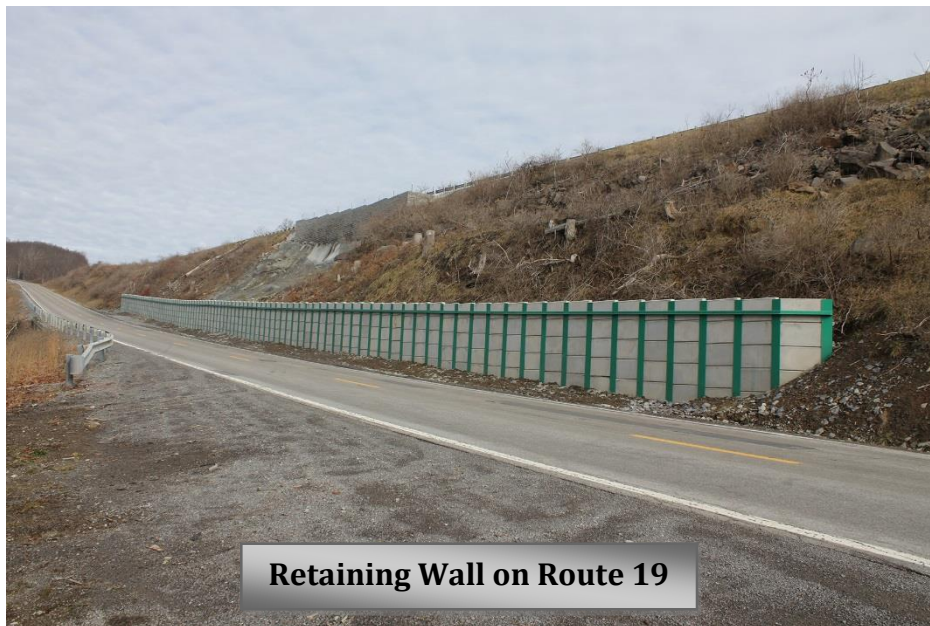
Mile 24 Southbound Slide Repair
