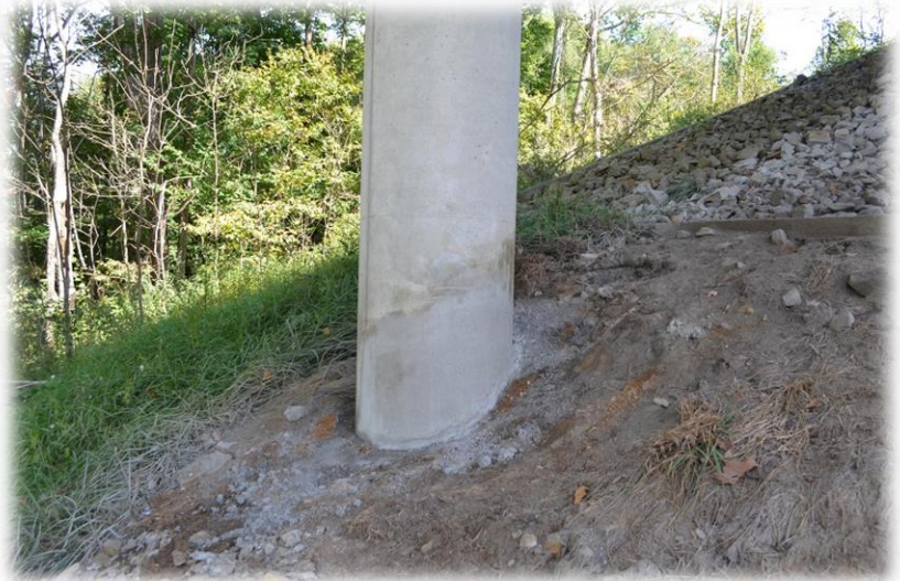
Pier Shotcrete Repair
