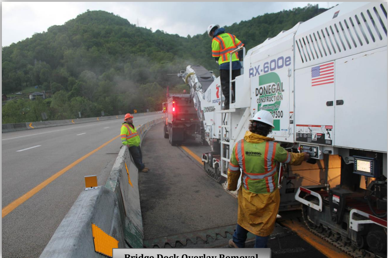
Bridge Deck Overlay Removal
