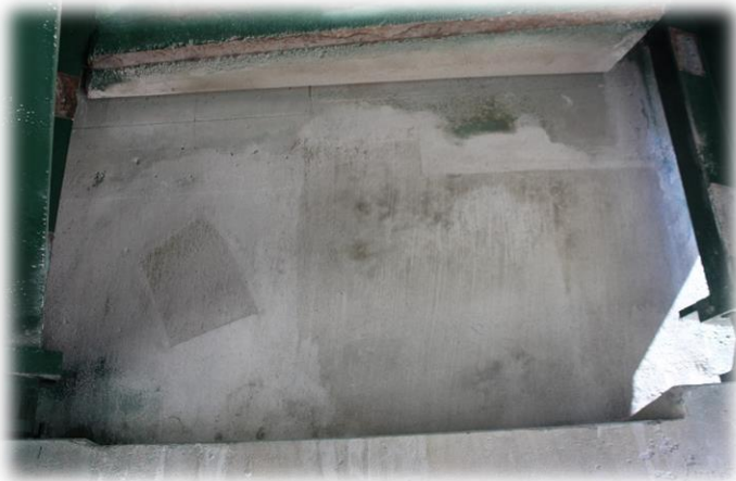
Delaminated Concrete Repaired on Backwall
