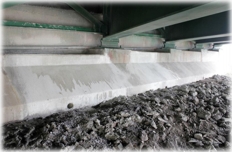
Abutment Shotcrete Repair
