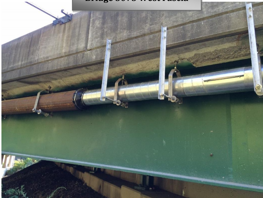
4" Waterline Installed On Bridge 3073 West Fascia
