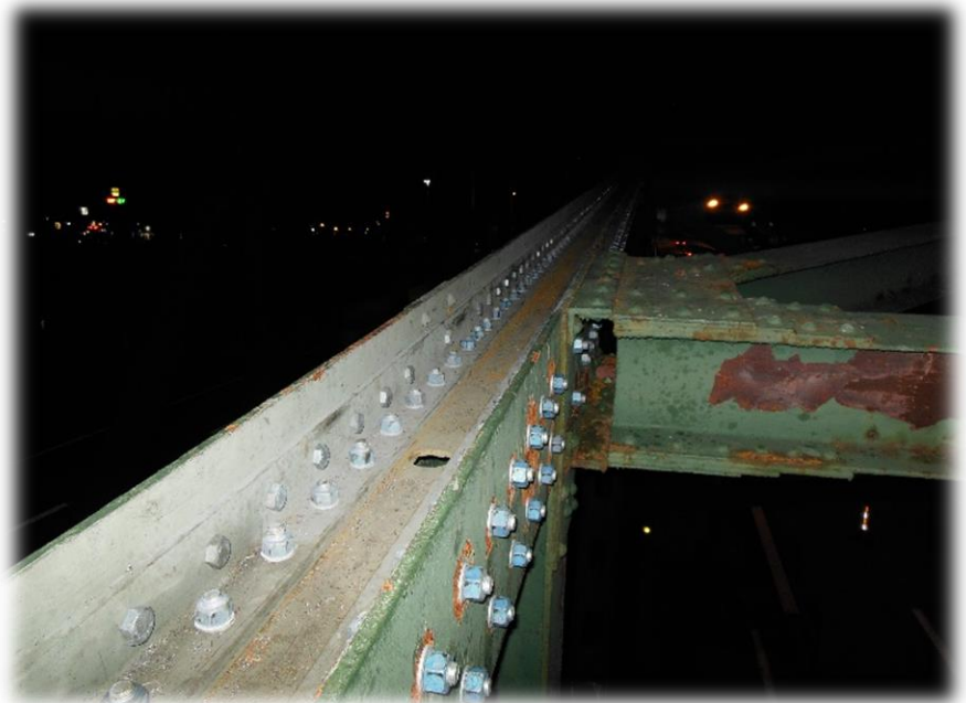
Longitudinal Angles Installed on the Top Chord of South Yeager Bridge
