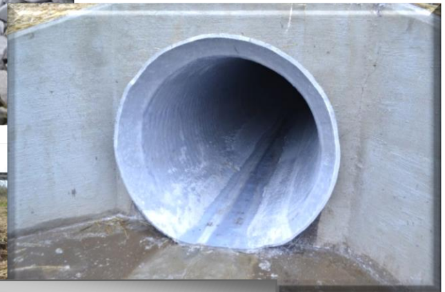
Insituform Pipe Repair
