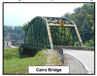
structural solution for a bridge with a substandard roadway width and will require design exceptions. As a result, a rehabilitation alternative was dropped from consideration early in the planning and design process.
