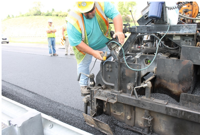
Figure 9: Angle adjustment by screed operator
