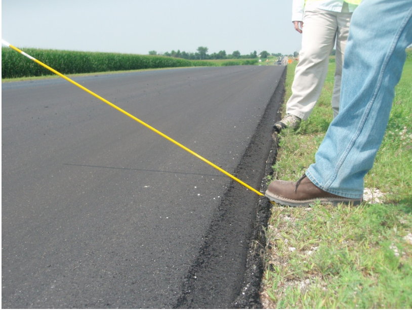
Figure 1: Typical Safety Edge SM installation
