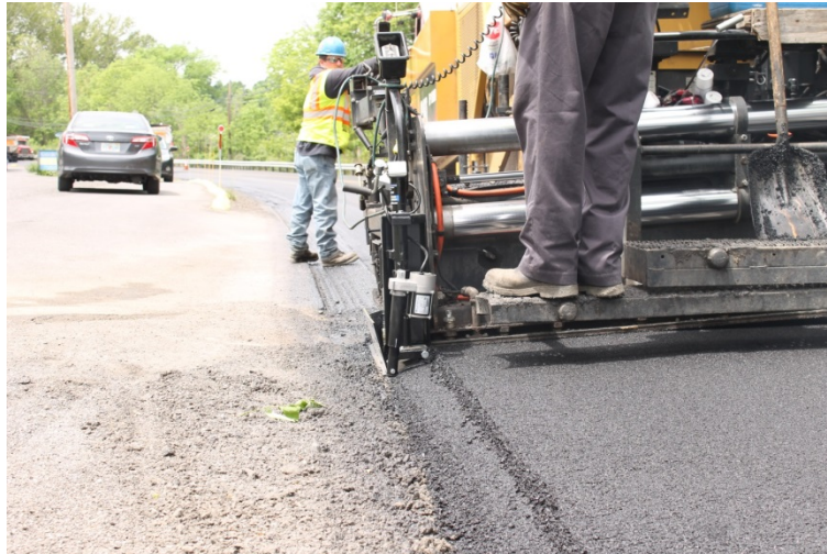
Figure 4: SE installation on SR 150
