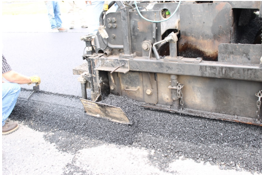
Figure 5: Measurement of SE before rolling
