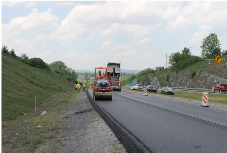
Figure 3: Paving operation on SR 322
